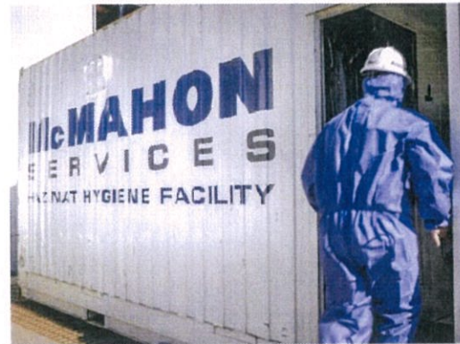
Figure 7: Image shows an external fully contained 2 shower decon unit
