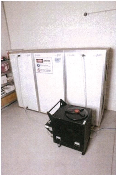
Figure 6: Image shows the portable 2 shower decon unit with adjoining water filtration unit
