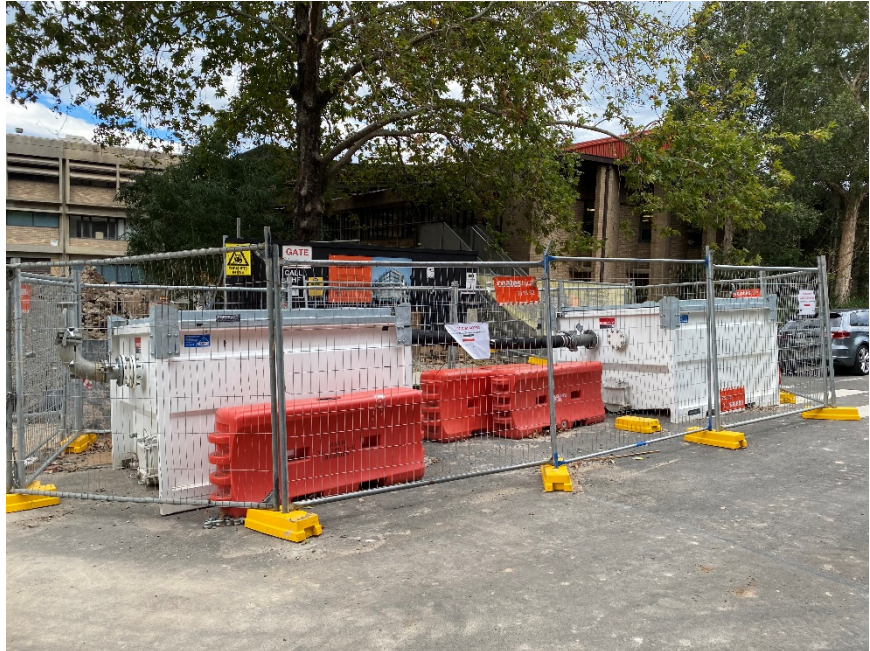
Photo 4: Stormwater storage tanks for testing prior to disposal.
