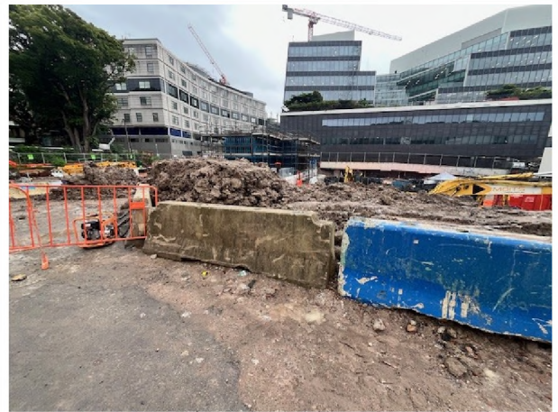
Photo 1&2: Heavy vehicle site access barricaded off due to wet weather stop works. Purple Cow skip bin. Stockpiled material for future reuse or load-out.
