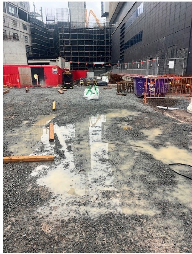
Photo 17: REF stormwater works were complete
