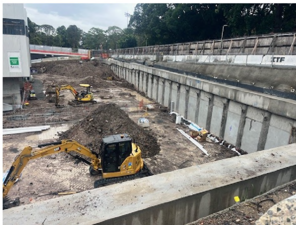
Photo 9: Piling and capping beams were complete
