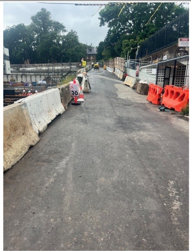
Photo 4: Heavy vehicle access stabilised and no signs of tracking along the access.
