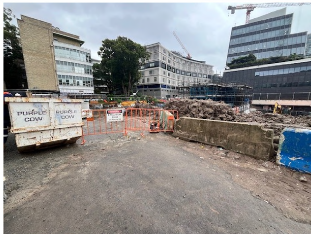
Photo 1&2: Heavy vehicle site access barricaded off due to wet weather stop works. Purple Cow skip bin. Stockpiled material for future reuse or load-out.
