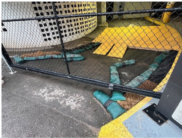
Photo 13 & 14: ERSED controls around stormwater inlets near the site compound were maintained in good condition
