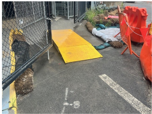
Photo 13 & 14: ERSED controls around stormwater inlets near the site compound were maintained in good condition
