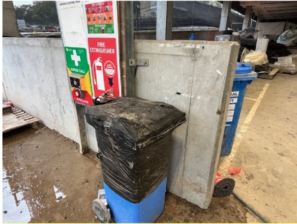
Photo 11: Spill kits were provided but signage was missing (covered with black plastic)
