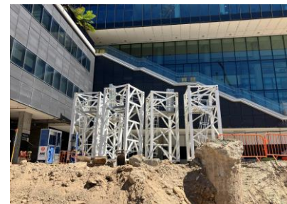
Image: assembly area setup for Tower Crane 2
