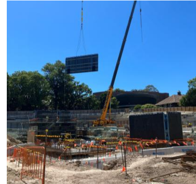
Image: First external jumpform shutter lifted into place for Core 3
