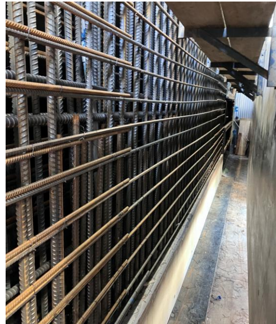
Image: inside look of the steel reinforcement internal to Core 2
