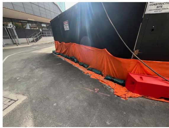
Photo 16 & 17: ERSED controls established and maintained in good condition around the base of the hoarding on the low side of the site (near entrance to the undercroft)
