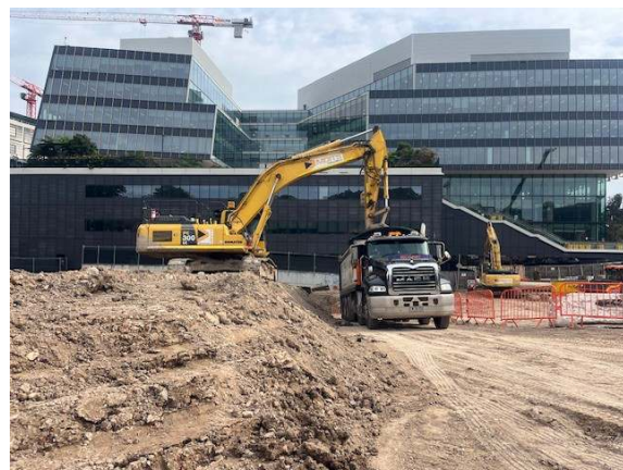
Photo 19: Spoil load-out was underway from the main stockpile
