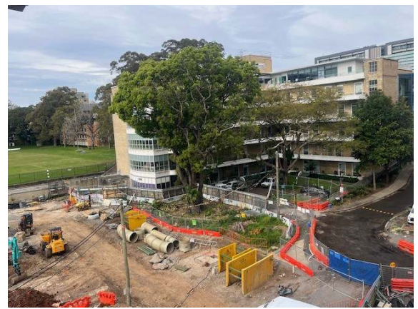
Photo 15: REF stormwater works and tree protection zone established
