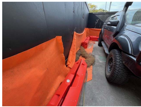
Photo 16 & 17: ERSED controls established and maintained in good condition around the base of the hoarding on the low side of the site (near entrance to the undercroft)
