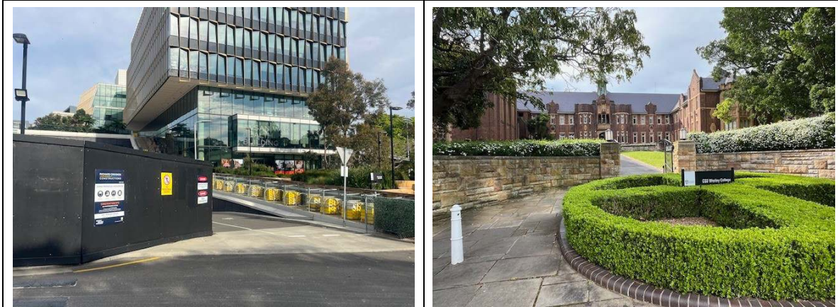
Photo 3: Susan Wakil Health Building (SWHB) to the north of the site
