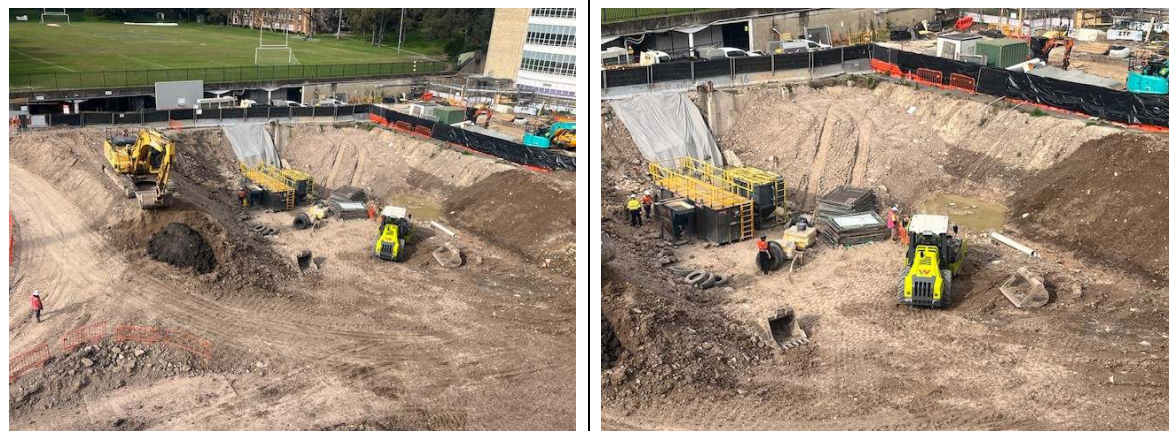
Photo 10 & 11: Set-up of the hazardous materials exclusion zone, including asbestos fibre air monitoring
