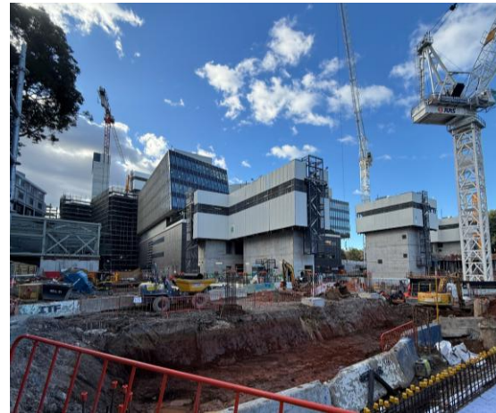
Image: Ongoing stormwater culvert works
