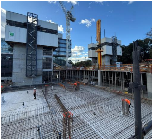
Images: reinforcement and formwork activities across Level 1 and Level 2
