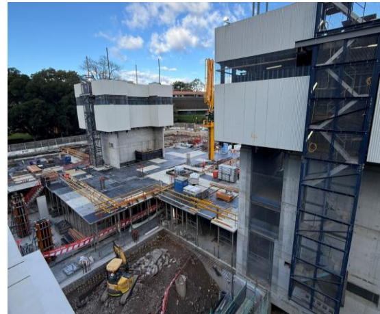
Image: Suspended slab pours at Level 2 between Core 2 and 3
