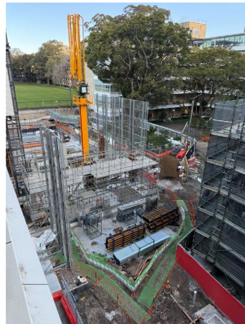
Image: Building B starting to take shape with scaffolding and screen installed in advanced of concrete pours
