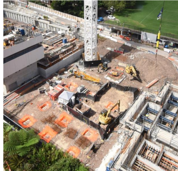
Image: Contained hazmat work area between Core 1 and 2
