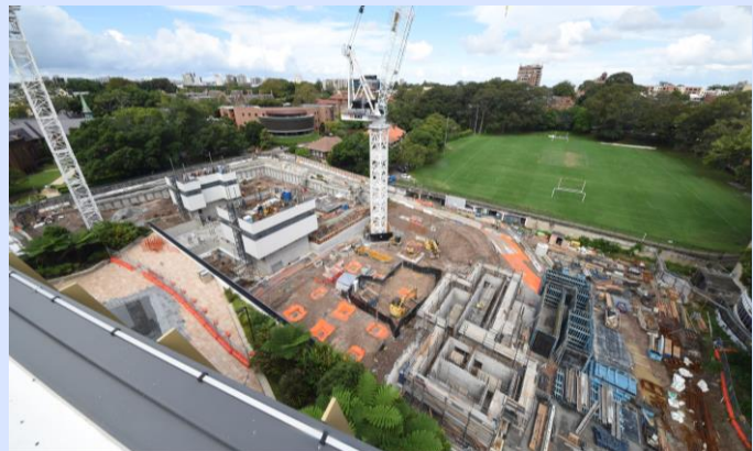
March 2026 – Substructure underway and foundation piling complete
