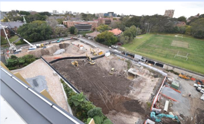
July 2025 – Retention and foundation piling and bulk excavation commencement
