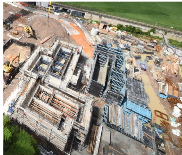
Image: Core 1 base wall and jumpform assembly ongoing
