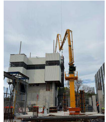
Image: Tower Boom Pouring Concrete into Core 1
