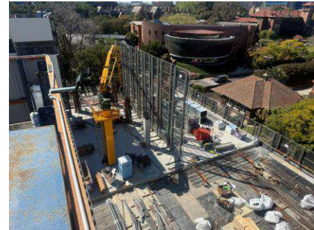
Image: First Level 4 Slab poured
