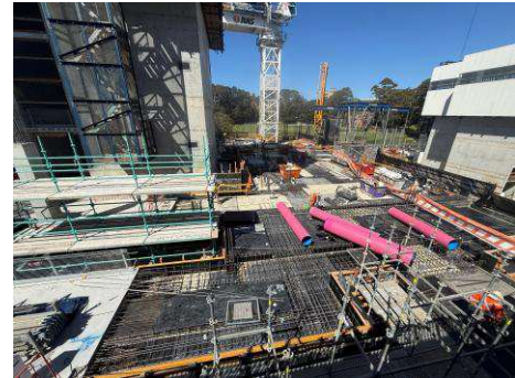
Image: Level 03 Reinforcement being installed
