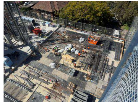
Image: L4 deck completed / Column Prefabrication Area
