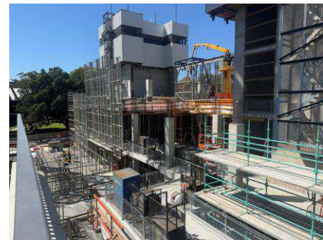
Image: Protective screens climbing higher
