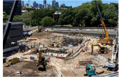
Image: Core 2 and 3 progress of substructure
