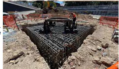
Image: Tower Crane 2 base preparation works
