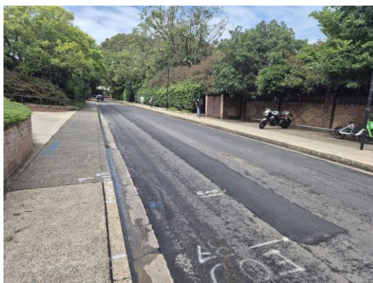
Image: Western Avenue reinstated after excavation works for future HV
