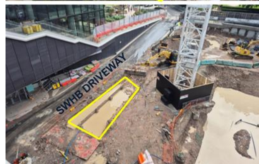
Image: localised exclusion zones for hazmat removal works
