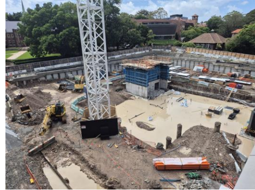
Image: site clean-up ongoing , including de-watering and water treatment, due to large rainfall over last weekend.
