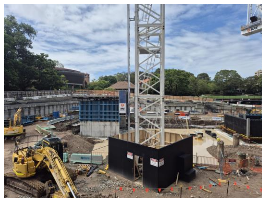
Image: security measures installed for Tower Cranes incl. 3m hoarding at base
