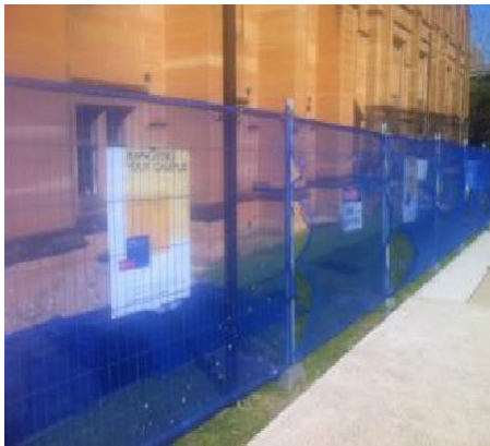
Image 3 - Fencing with Cloth and Signs
