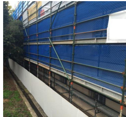
Image 4 - Scaffold with Hoarding and Cloth
