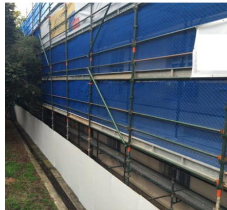
Image 4 - Scaffold with Hoarding and Cloth
