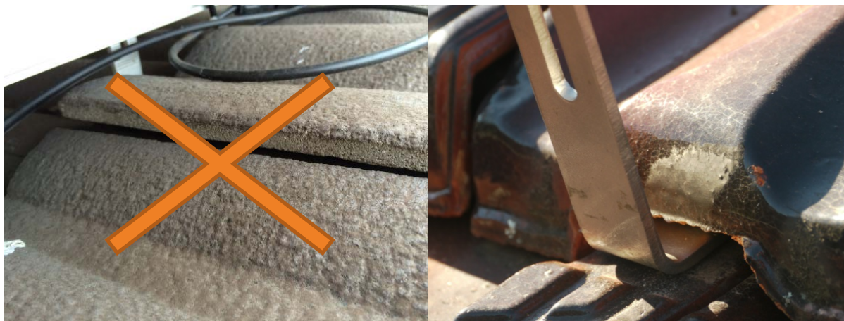
Figure A8.1. Left: incorrectly installed tile hook without grinding tile. Right: correctly installed tile hook with ground tile so that the tiles can lay flat.
