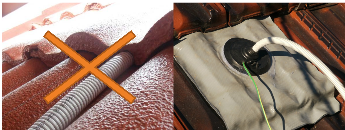
Figure A8.2. Left: wiring system penetration incorrectly installed between tiles. Right: wiring system penetration correctly installed with vertical penetration using a collar flashing.
