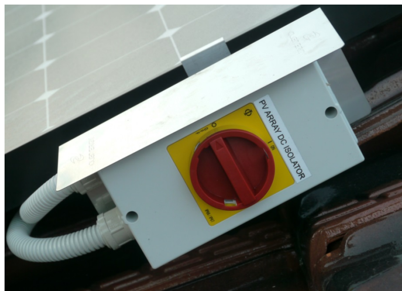
Figure A5: Shroud installed over rooftop isolator at the array
