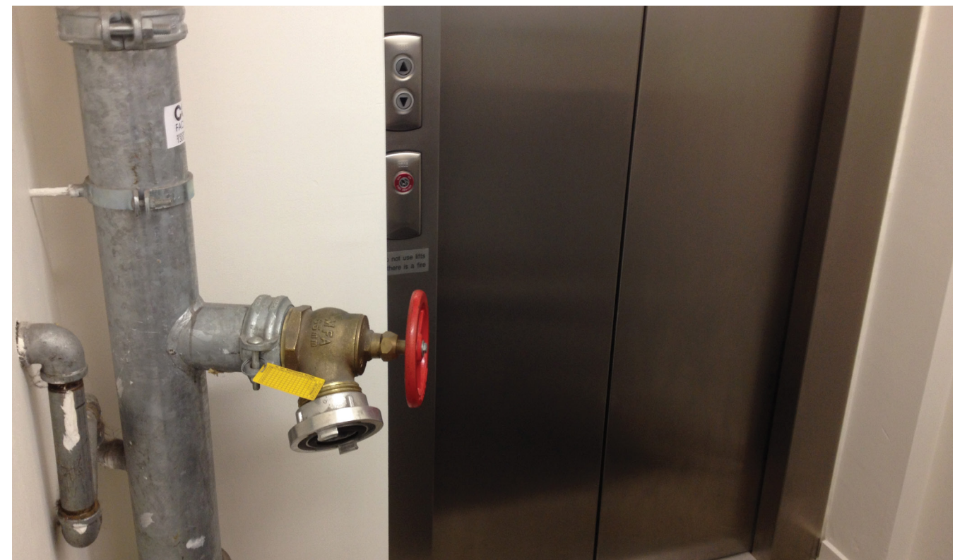
Fire hydrant adjacent to lift (cannot be taken up or down floors from this point, must be near a stair) in an 8 storey building. Nearest stair 25 m away.
