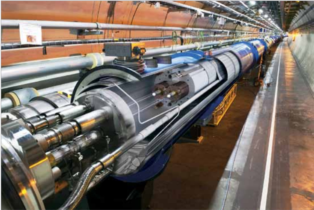
Figure 15. Photograph of the LHC collider installation, with illustrated cut-away showing the particle beams.
