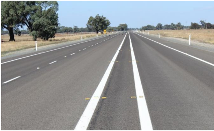
Wide centre line and shoulders on the Newell Highway in southern NSW
