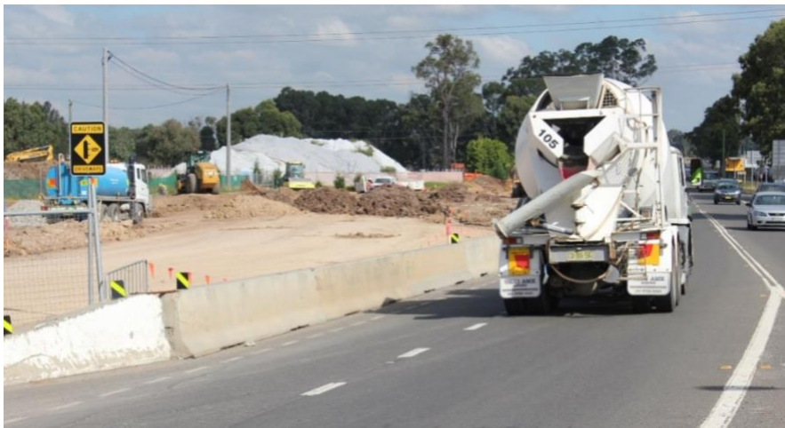
Parts of The Northern Road upgrade
