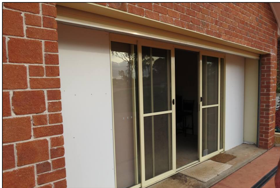
Figure 11: Conversion of a garage to an unauthorised dwelling, via removal of a garage door
