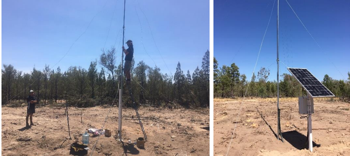
Figure 1: LoRaWAN Tower being installed on Llara Farm which provides coverage in a 10km radius. It is a long range low power wireless network – March 2018
