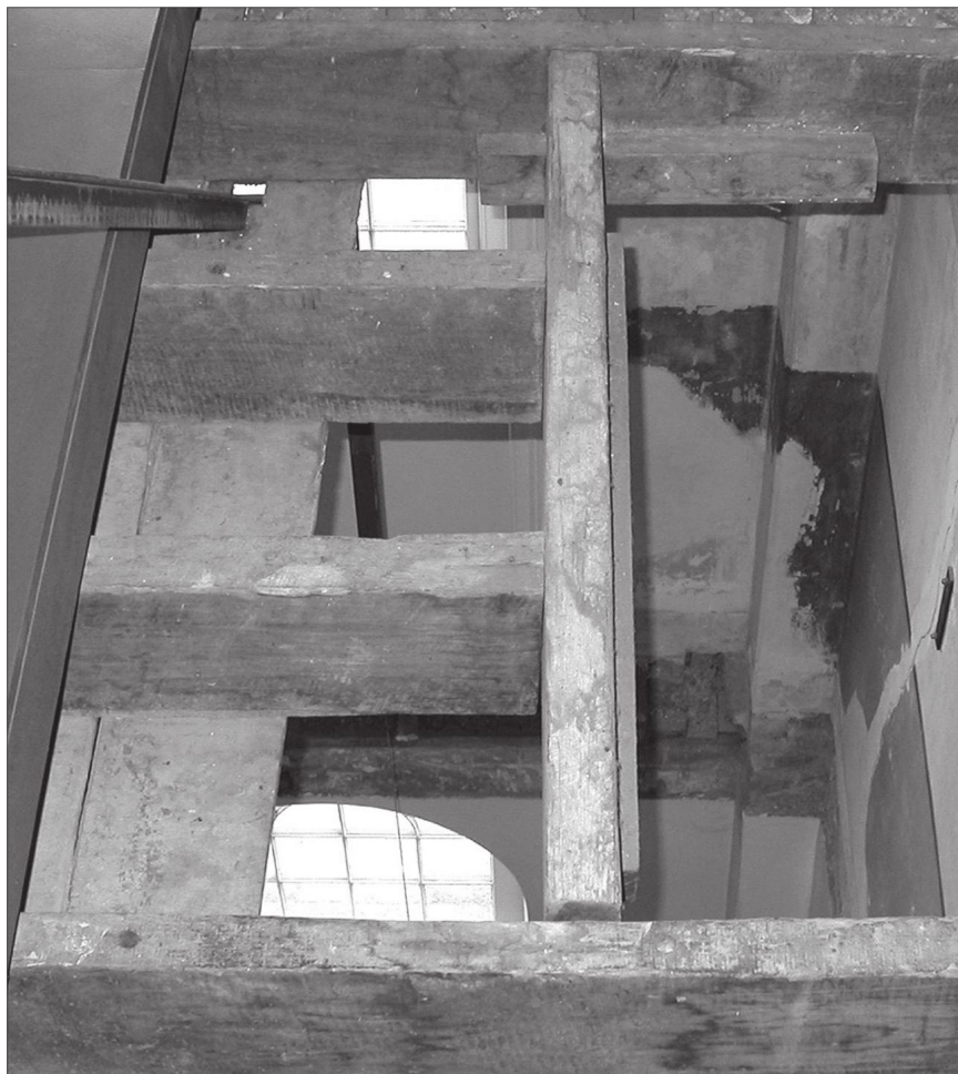
Figure 2.3: Floor cavity on Level 3 (P. Davies 2009).
