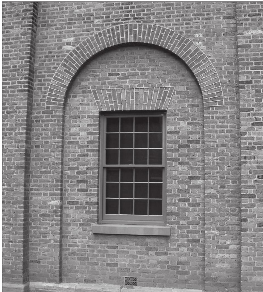
Figure 1.5: Detail of Level 1 window (P. Davies 2008).
