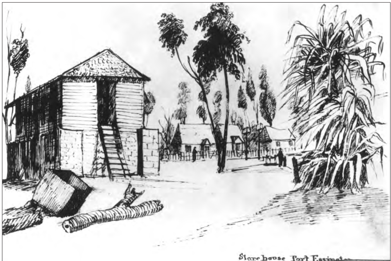
Figure 110. Quartermaster's Store, looking east. Note the original piles had been encased in stonework when this drawing was done, dating it before 1843. Watercolour by Owen Stanley, entitled Storehouse Port Essington . Mitchell Library PXC 281 f.63b. Published with permission of the Mitchell Library.
