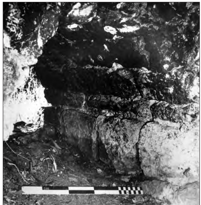
Figure 54. Entrance to kiln no. 3 from within, showing thickness and construction of walls.
