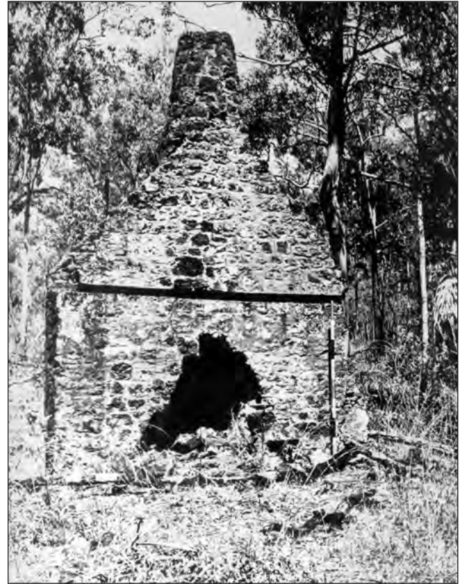
Figure 19. Married Quarters round chimney no. 4 showing horizontal beam revealed on internal face.
