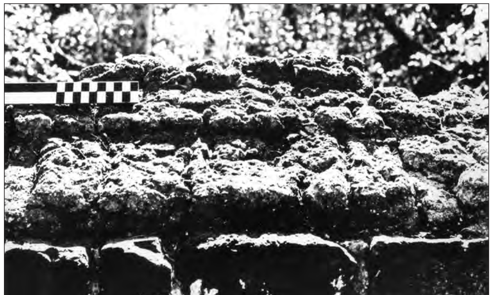
Figure 40. Detail of bakery roof. Impressions in the cement suggest the roof was originally covered with wooden shingles.
