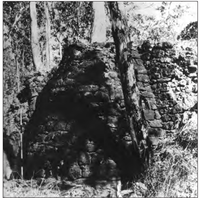
Figure 53. Kiln no. 3 showing how it was built into the 4 metre high bank and protected with a retaining wall on each side. The lower entrance to the kiln is in the shadow of the tree.
