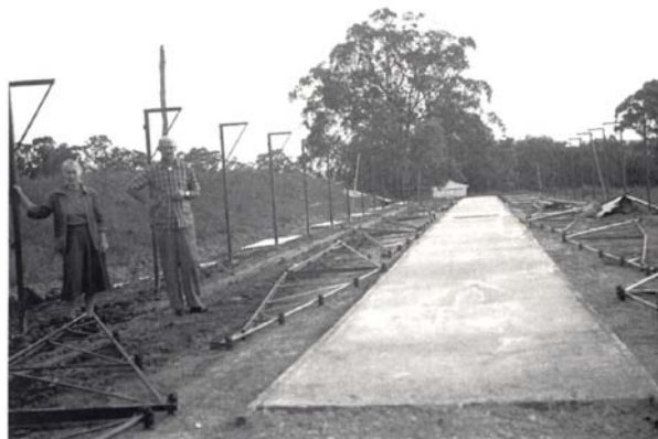
Construction of the first layer shed 1959 (Dr. Harold McNary & Mrs. Janet McNary)
