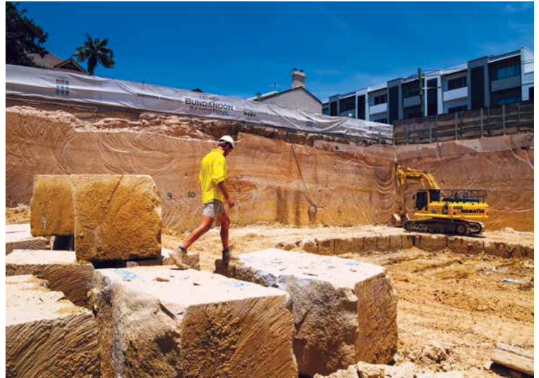
▲ Digging deep in Pymont. When buildings come down, crews move in while they can, to grab more sandstone for maintaining the historic buildings of Sydney. Kennerley / Sydney Morning Herald
